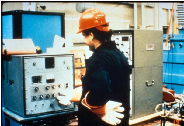
Fig.1: Capacitance and dissipation factor bridge (manual balancing method).
