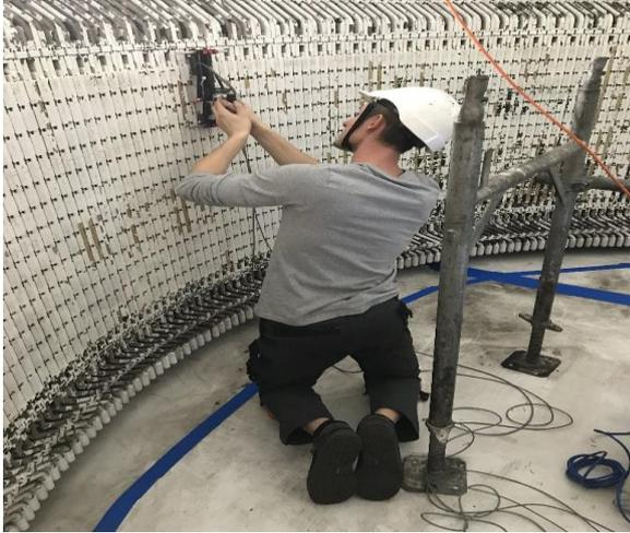
Fig. 8: Scanning of stator core with search coil
